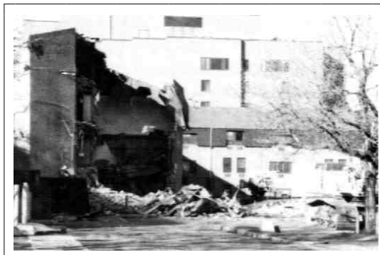
Cooney Hall, mid-demolition
